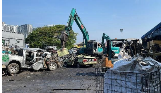
Dismantling Using Nibbler
