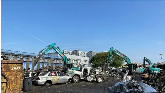
Final Dismantling Area
